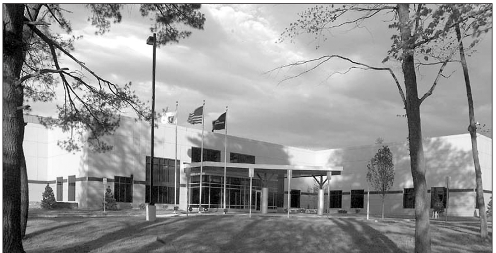
The American Superconductor building in Devens was a perfect example of design-build. Final design of the warehouse area was on hold while the equipment went through a number of redesigns, but construction continued in other areas of the facility.
