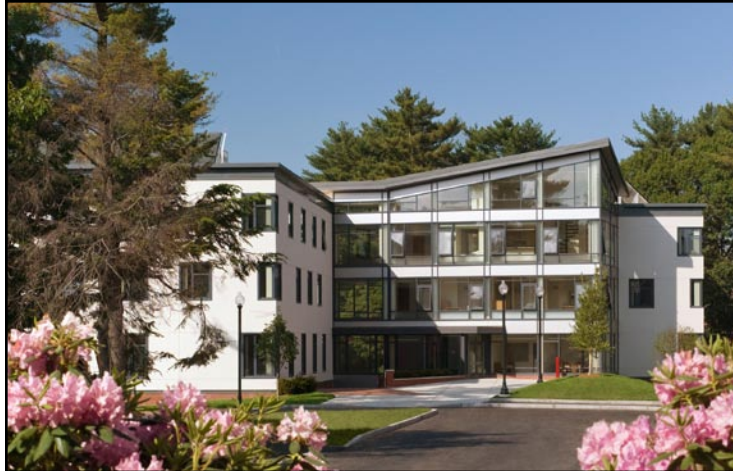
Mount Ida College's new residence hall features a "pod" design that combines the best elements of traditionally-programmed dormitories while fostering interaction and community building among students. (Photo credit: Anton Grassl/Esto)
